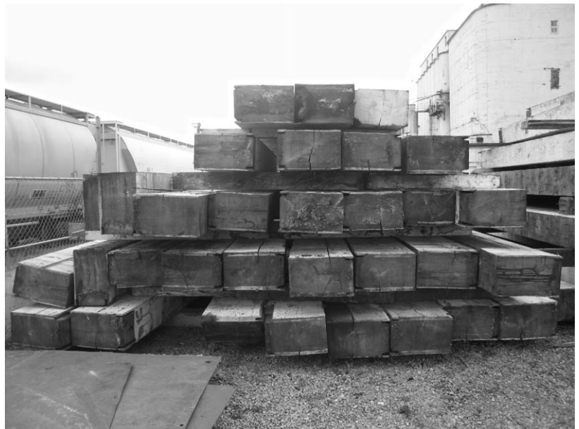
20-ft. 16x24-in. timbers stacked neatly at the deconstruction site.
