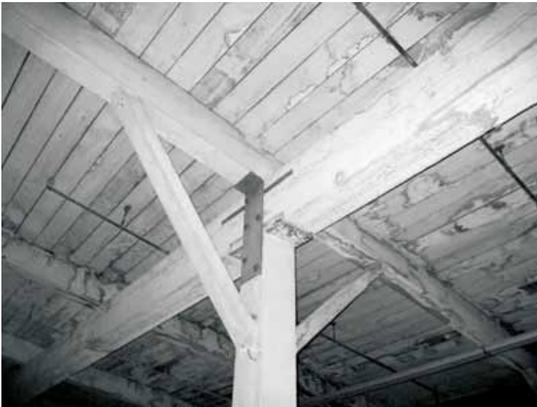
Post-beam junction in a 1905 warehouse.
