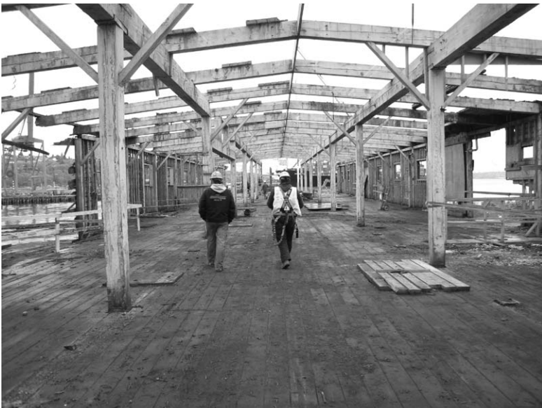
Deconstruction in progress showing roof framing and decking in a 1905 warehouse.
