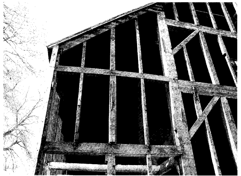
Photos and drawings Jack A. Sobon Sheathing direction determines the orientation of wall framing. This early 1800s barn (now dismantled) from Middleburg, N.Y., has studs to support wide clapboards. Note how the braces take precedence over the studs.
