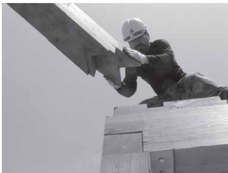
Mr. Soonho Hong guiding a timber into place.
